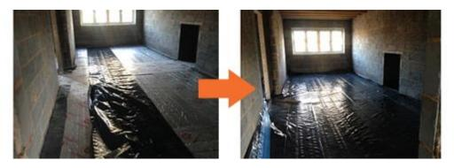
**Step 4**Perimeter insulation should be fitted around all walls (also over the 500 gauge membrane if applicable). If using liquid screed, pull the plastic skirt out and tape the skirt to the membrane. Tape all joints in the membrane. See pictures below.
