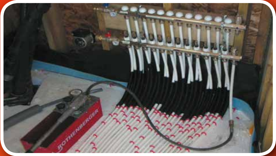
Figure 3 - using a test pump to pressurise the system to 5 bar
